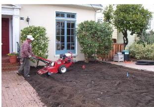
Most of the time the natural soil inside the rain garden needs to be amended. Depth of amended soil varies from 1.0 to 2.5 feet.
